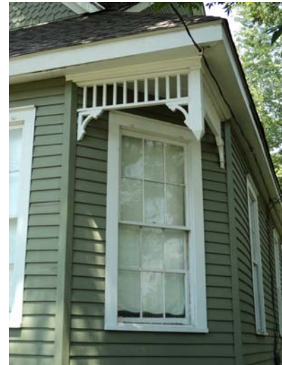
This double hung, wood window is a character defining features that includes the historic glass and some Victorian “gingerbread” detailing. Olde Towne, Slidell, 2011
