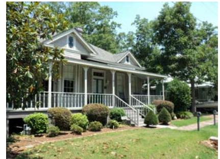
Wood spindles, columns, shutters, and window elements on a Victorian house in Olde Towne, Slidell, 2011.
