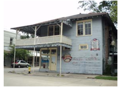
This historic building in Olde Towne includes wood siding, wood gallery elements, exposed wood rafters, and wood window and door trim. Olde Towne, Slidell, 2011
