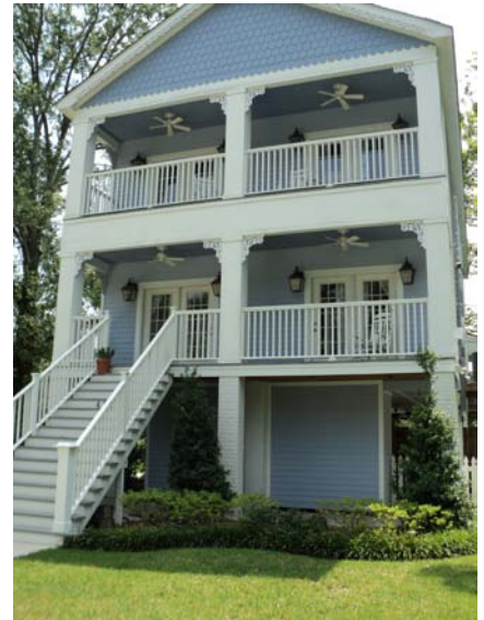
This new construction is a 3 story building due to the new building height and BFE requirements, and uses features and materials that are compatible with Olde Towne, Slidell. 2011.
