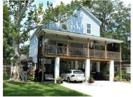
The rear façade of a new construction Project in Olde Towne, Slidell that includes a raised foundation; parking is obscured from the street with a breakaway wall. 2011.
