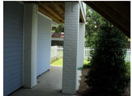
CMU columns with brick veneer on a new construction project with a raised foundation in Olde Towne, Slidell, 2011.
