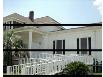
This ramp includes a simple, painted wood balustrade or railing that makes the ramp appear appropriate for the style of the historic building. Olde Towne, Slidell, 2011
