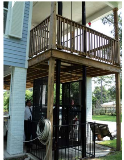
An elevator addition on a new construction project in Olde Towne, Slidell; elevator is appropriately located at the rear façade, and includes materials that are compatible with the historic district. 2011.
